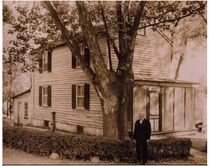
George Arrowsmith, last bridge tender, stands in front of Port Mercer Canal House
